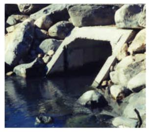
SRICD successfully led the effort to replace an old 18-inch culvert (shown at left) with a 3x4-foot box culvert (shown at right). The new culvert restores tidal flushing, which in turn, is eradicating exotic invasive plants and allowing the return of native marsh plant communities to Duck Cove.
