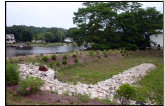
“This innovative treatment system at Mettatuxet Beach in Narragansett incorporates both infiltrators under the parking lot (top) and the dry pond (bottom) to protect the Narrow River.”
