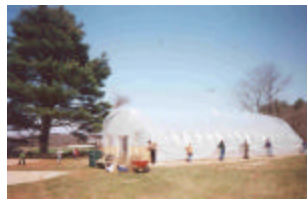
The RI Air National Guard constructs the new Kids Grow! Greenhouse.
