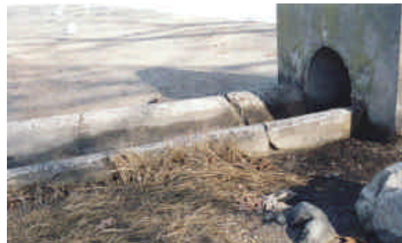
A storm water outfall in Narragansett.
