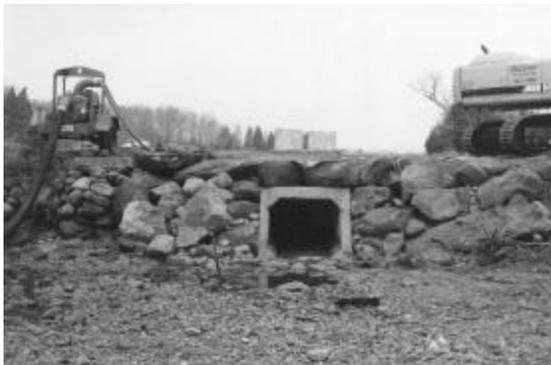
*Here's the new culvert shortly after installation, before the tides were let back into the Upper Cove.*
